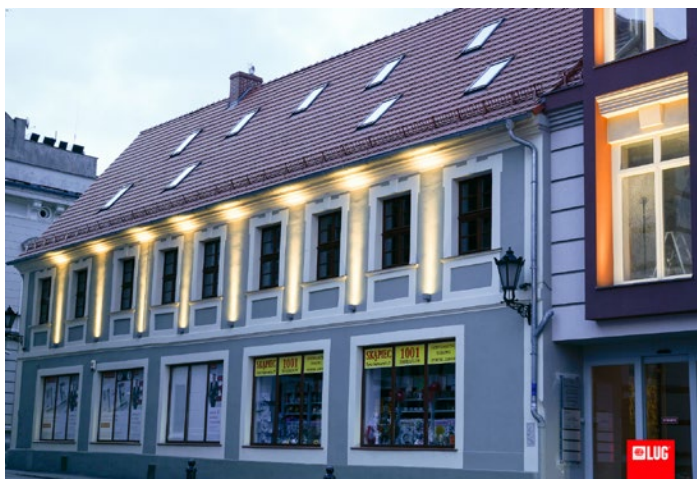
Tenant House in Mickiewicza Street, Zielona Gora, Poland
